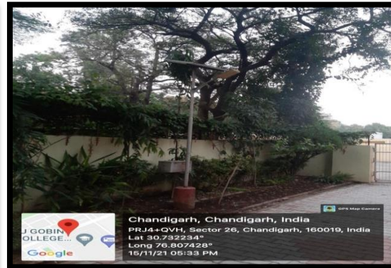
Solar Light in Boys Hostel
